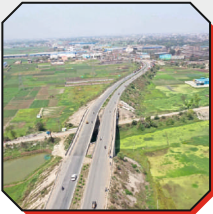
250 M WIDE 6 LANE EXPRESS HIGHWAY AHMEDABAD-DHOLERA
