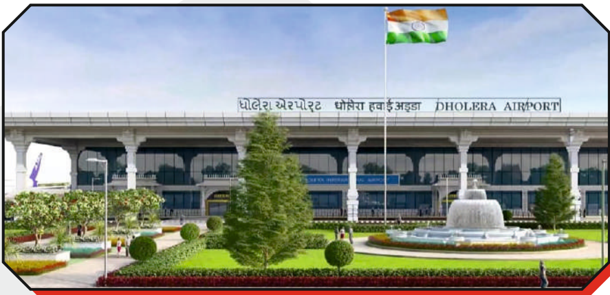
DHOLERA INTERNATIONAL AIRPORT
